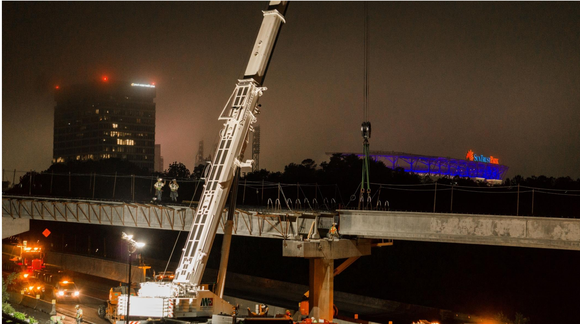
Nighttime beam setting at I-75/I-285 interchange
