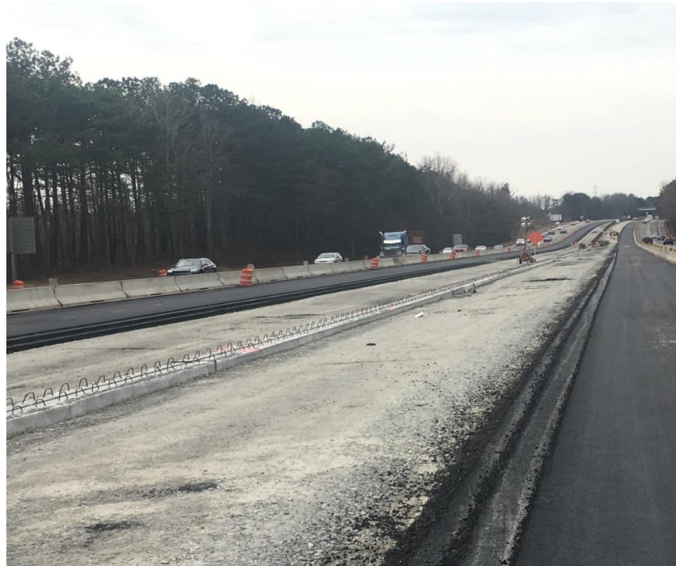
Asphalt paving and median barrier footing north of SR 20
