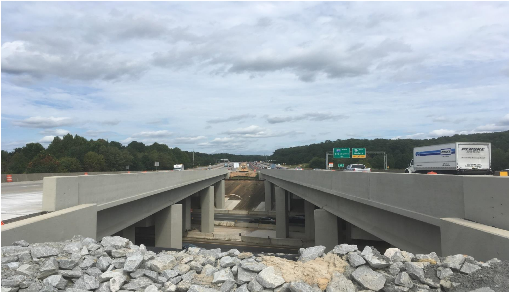
Newly widened bridge for I-85 Express Lanes
