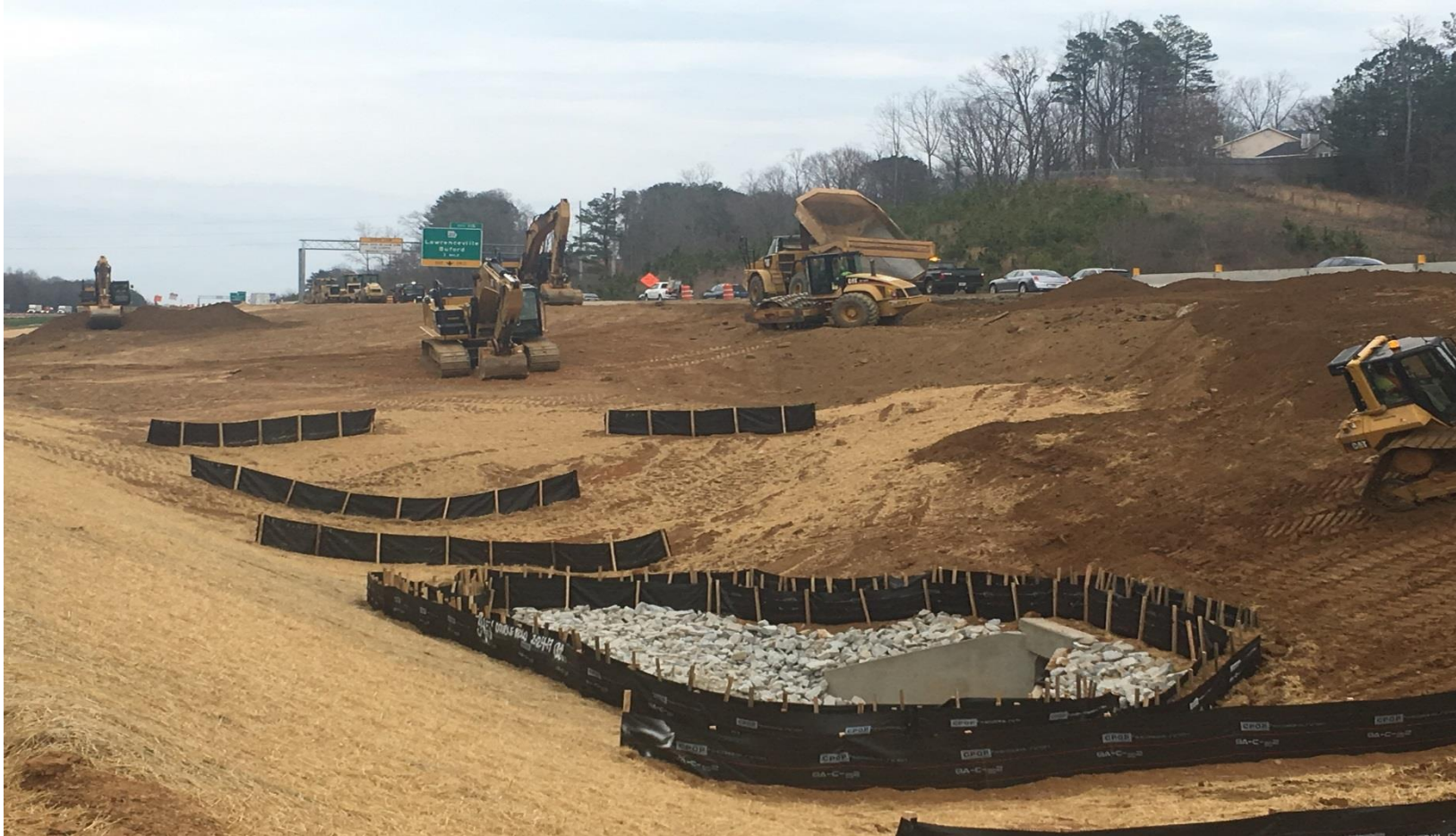
Median grading north of I-985
